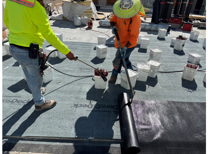
Palmer installing the new full re-roof near the central courtyard.
