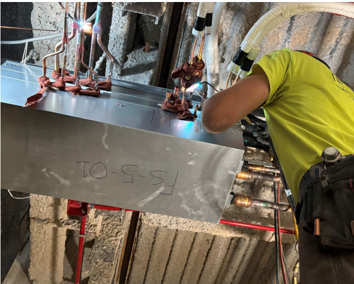
Total Energy Management brazing their refrigerant lines for the VRF system.
